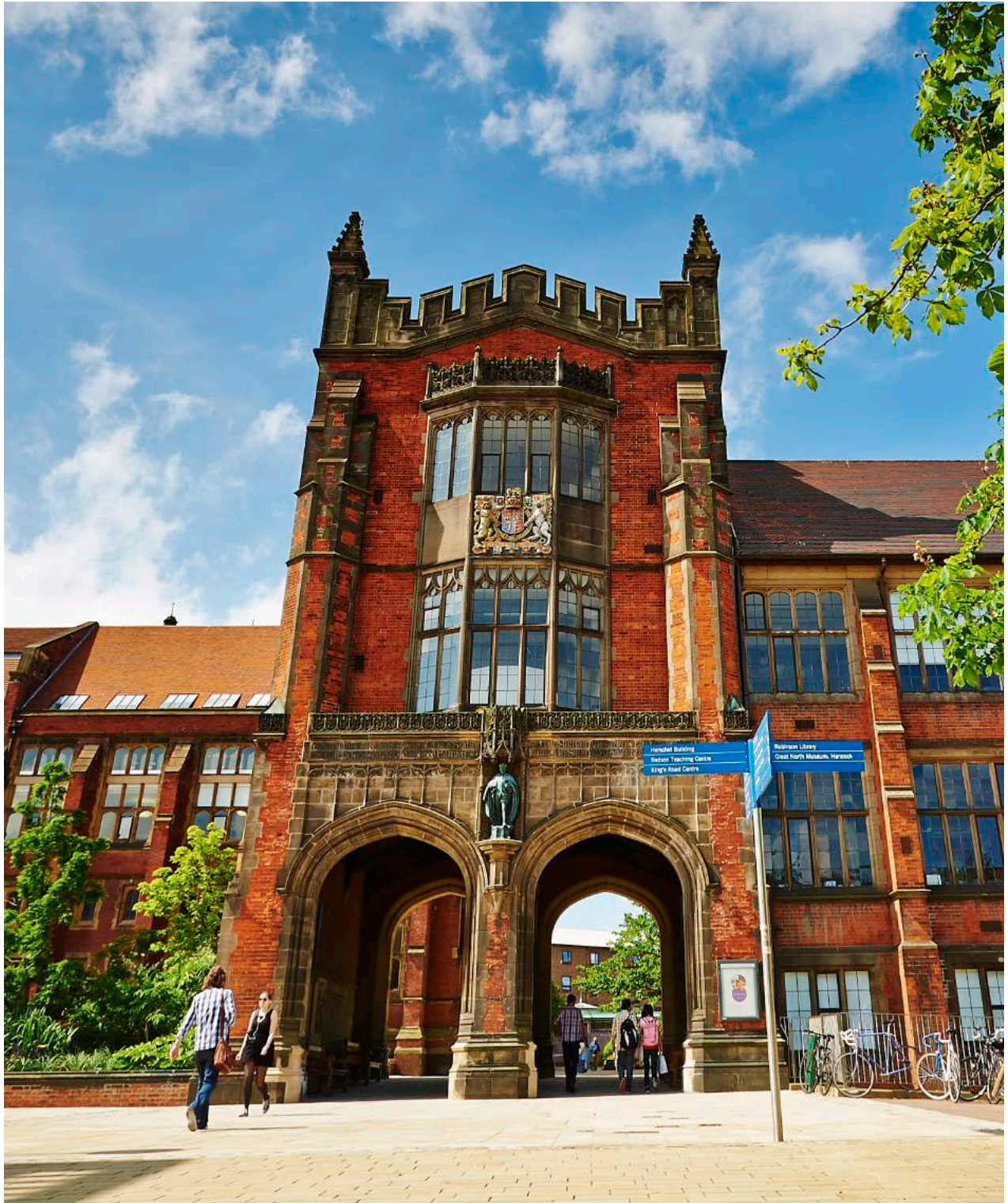
Arches on the main campus, Newcastle University, Newcastle upon Tyne
